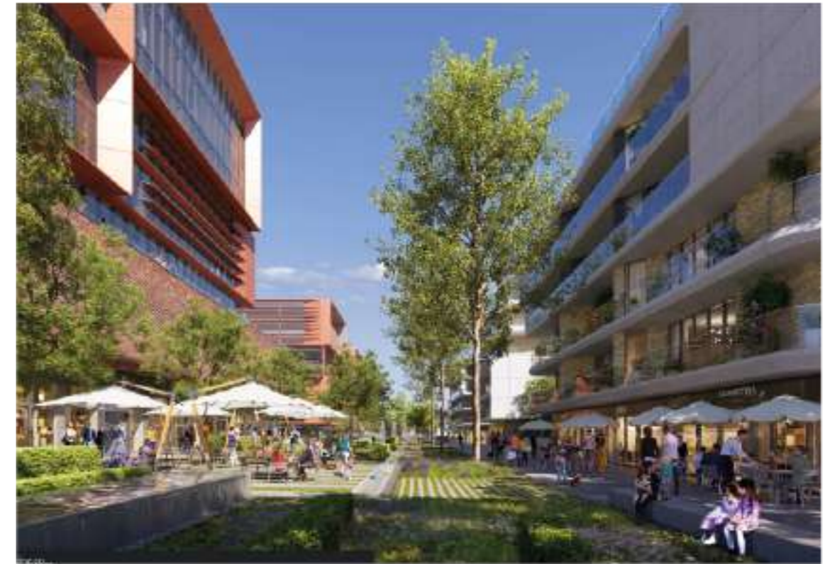
Zugló - Zaha Hadid Architects
