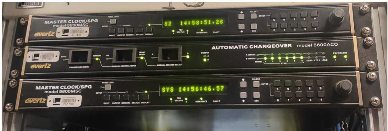
Figura 19 – Automatic Changeover model 56000ACO.
