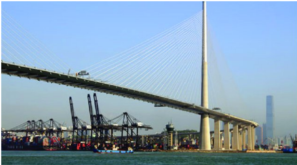
Figure 1.2: The Stonecutters Bridge in Hong Kong. Source: Research Gate, available at: https://www.researchgate.net/publication/335228501_Flexural_analysis_and_design_of_stainless_steel_reinforced_concrete_beams/figures?lo=1
