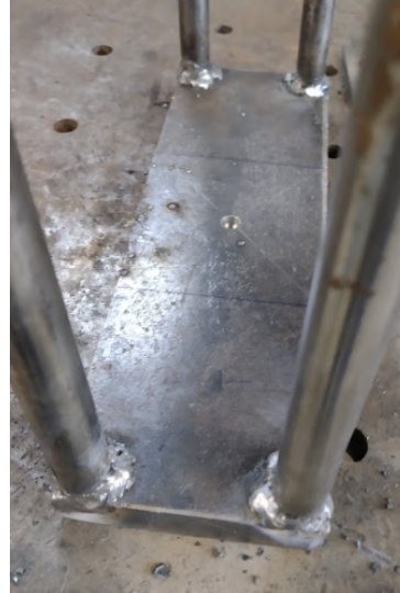
Figure 58 – Coated electrode weld applied between the plates and the bars.
