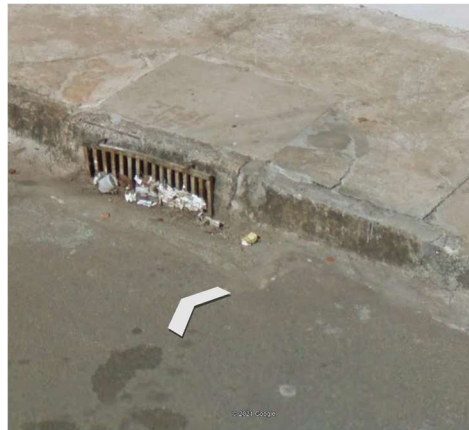
Figura 3.8 Boca de lobo com grades (Street View Google Earth, 2021)
