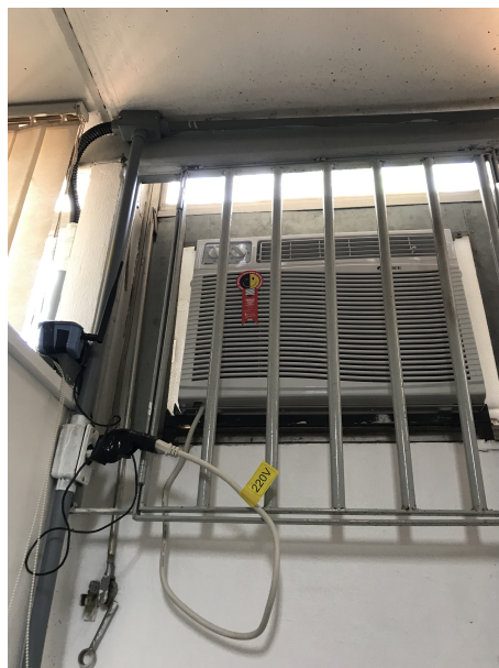
(b) Sensor instalado no GPDS.
