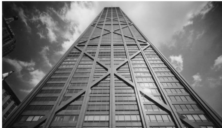
Figura 3.7: Fachada do Hancock Center, (Skidmore, Owings & Merrill LLP, 2019)
