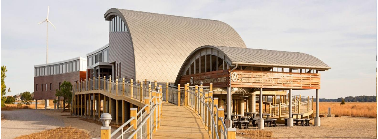
Figura 2.7 – Brock Environmental Center (Chesapeake Bay Foundation, 2014).
