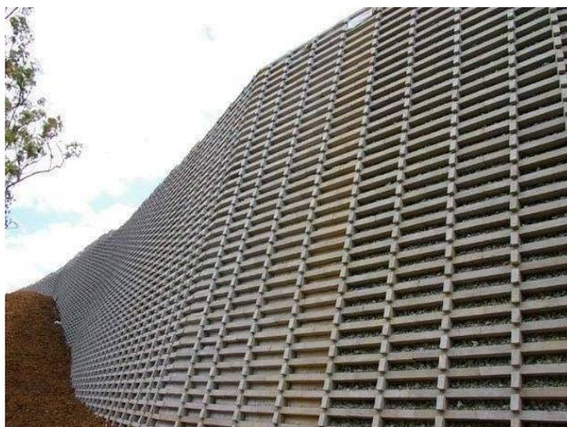
**Figura 2.6 – muro de *crib-wall*.**
