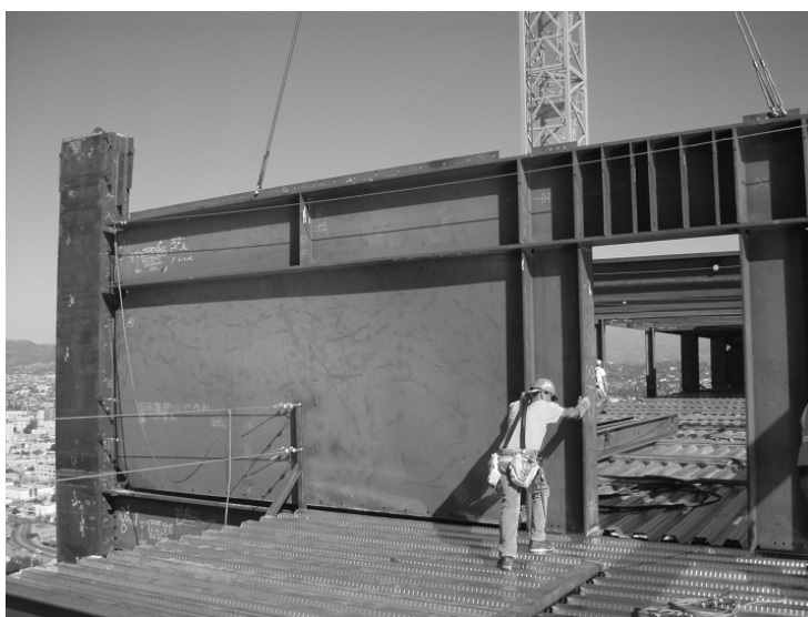
Figura 9 - "Steel plate Shear wall" (SPSW)
