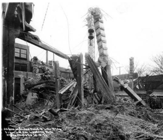
Figura 3 – Colapso do Prest-o-Building
